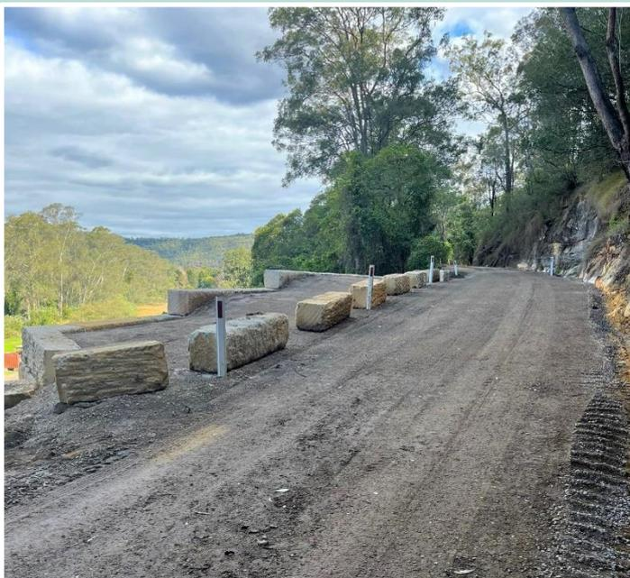
Retaining wall construction is now complete at both sites 1 and 2. Guideposts have been installed and drainage work has commenced this week. Jute matting will be laid below the sandstone walls next week to prepare for landscaping.
